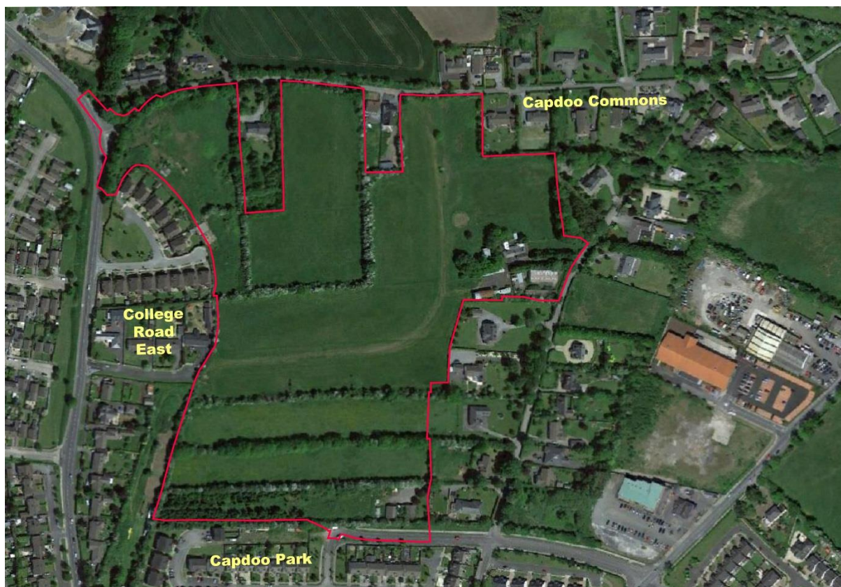
Fig 1.5 Aerial view of application site shown highlighted in red within the immediate context of the northern environs of Clane.
